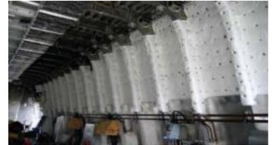
FireMaster Marine Plus used for bulk head
